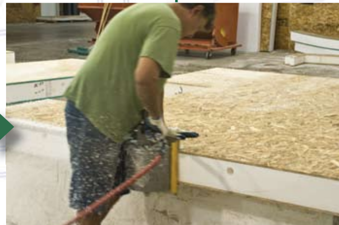
Operator using "hogger-style" cutting tool for cutting recess in EPS.
