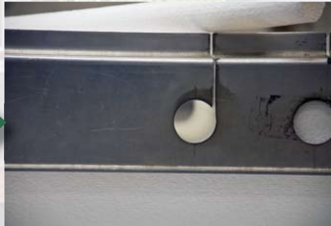
Finished cut for electrical chase.
